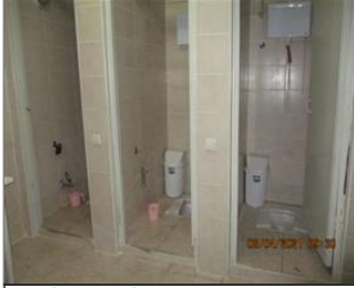
Photo of the sanitary facilities toilet (1).JPG
