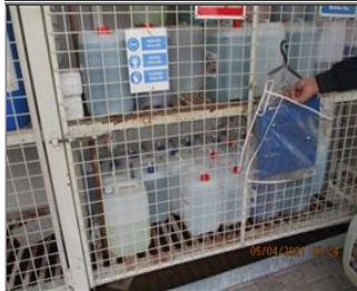
Photo of chemical storage room (if applicable) secondary containment available under chemicals.JPG
